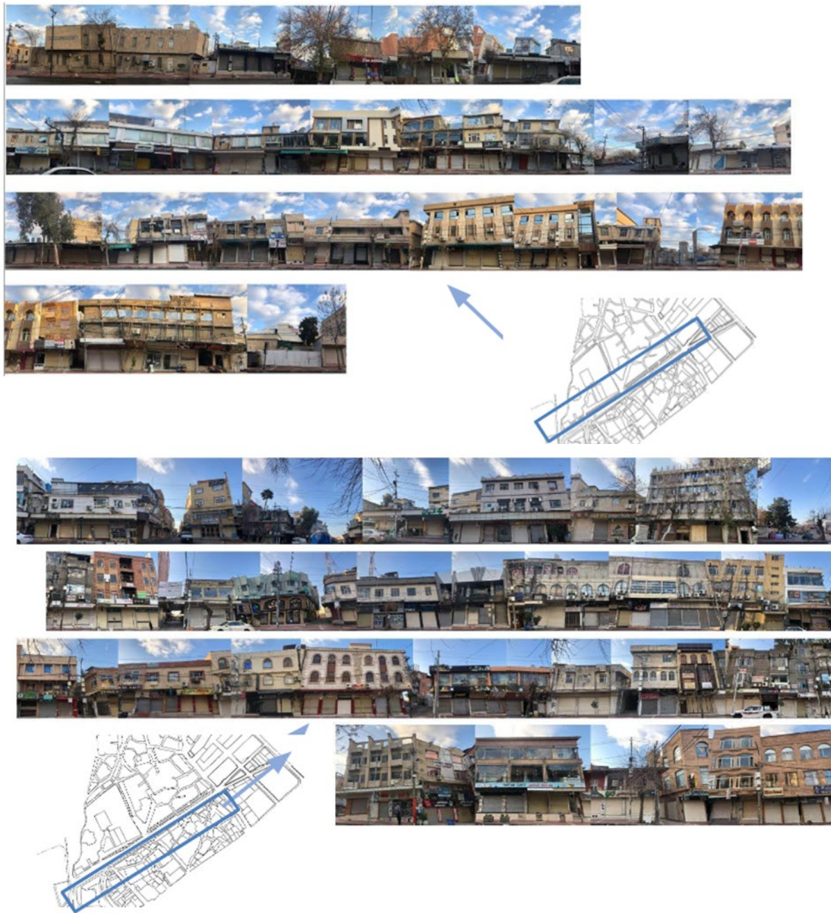
Figure 4: The skyline of both sides of Goran Street.
